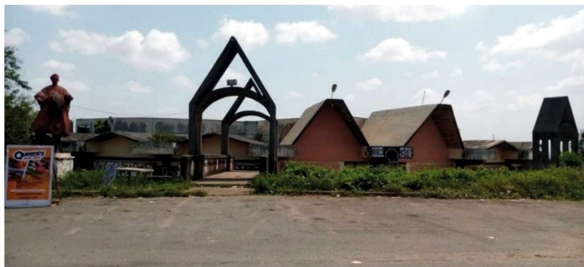
Figure (b): Exterior view toward the entrance of the Mokola cultural center showing sculptures of Yoruba music makers.
